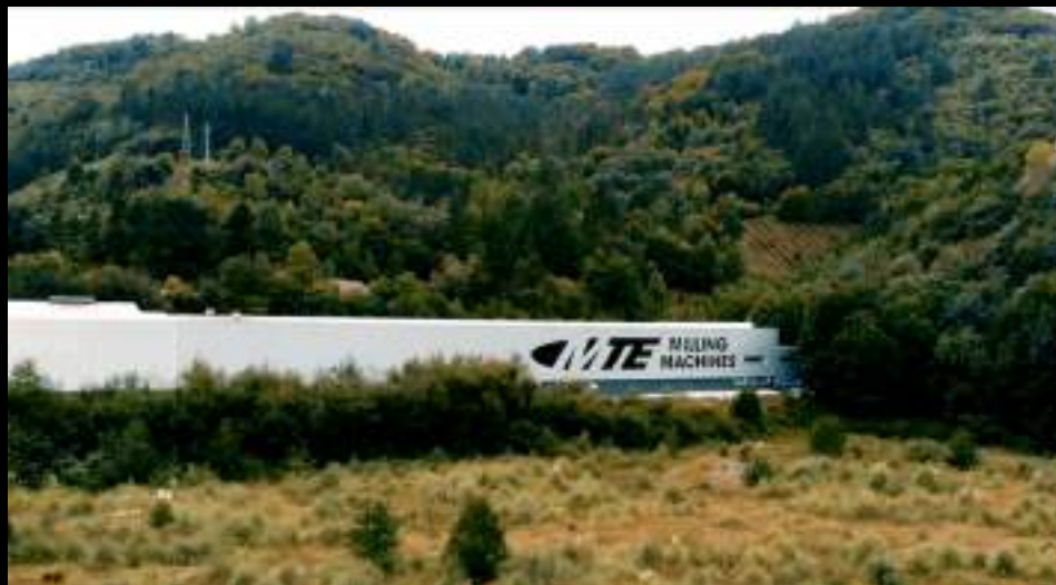
Headquarters Itziar, Gipuzkoa, Spain
